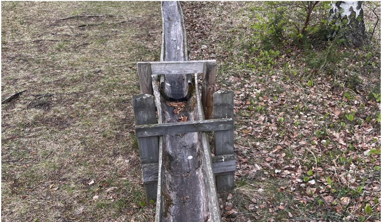
Example of part of the canal system, logs are often used for the last part of the irrigation system
